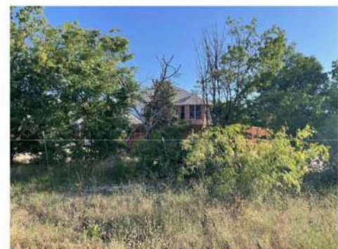
4 VIEW (EXISTING CONDITIONS)
