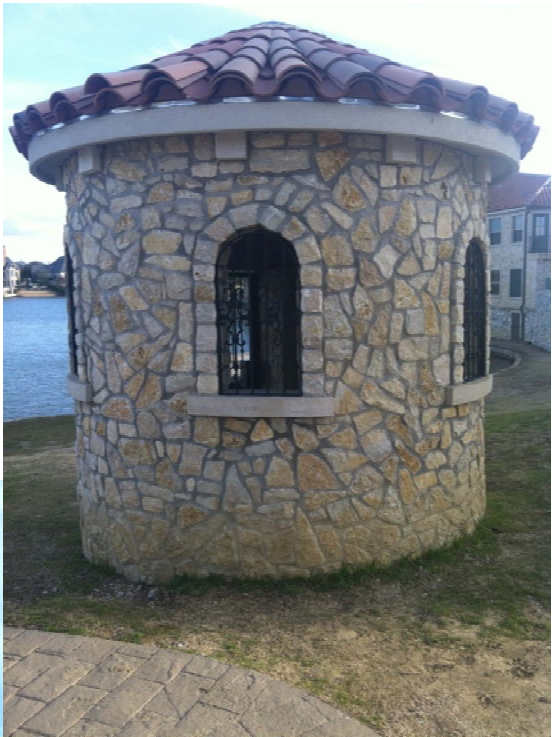
Right: a pavillion housing pump equipment for the lakes fountain
