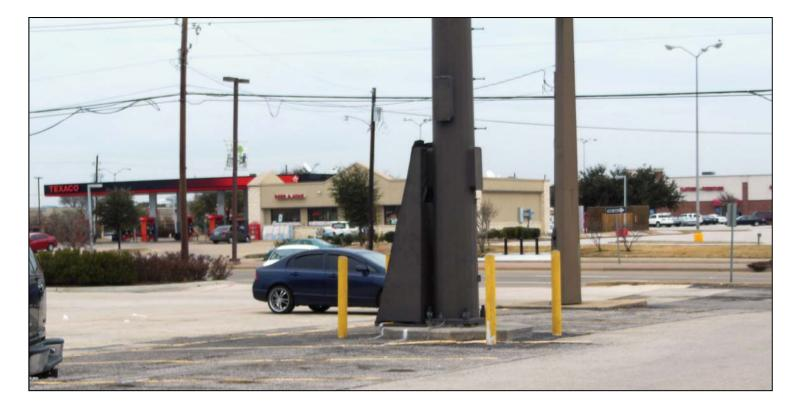
View of the Tower Base showing "Dog House". An additional "Dog House" (sloped structure to cover new wire conduit) will be added and painted to match the existing color.
